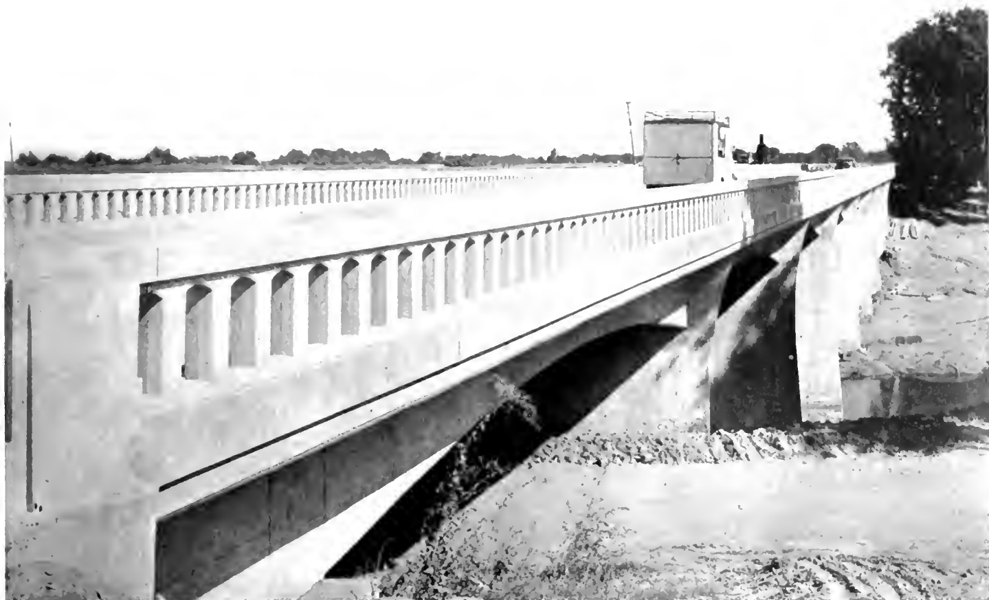
One of two one-way bridges on Davis-Dixon cut-off. Each one carries two lanes of traffic across Putah Creek
